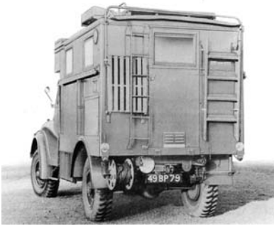
Note frame at top that folds down to support part of penthouse. A platform and ladder are carried at the rear.
